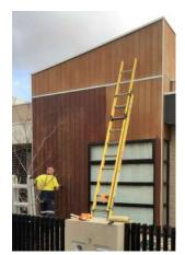
STAINING: Stain in the same direction that the boards run ea. Vertical for vertical cladding.
